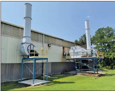
Viron Air Scrubber and Tri-Mer Blower Fan
